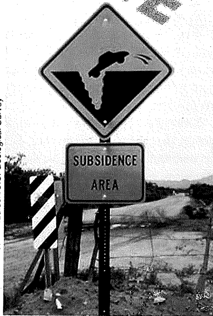
Sign warning motorists of subsidence hazard was erected after an earth fissure damaged Snyder Hill Road in Pima County, Arizona, 1981.
